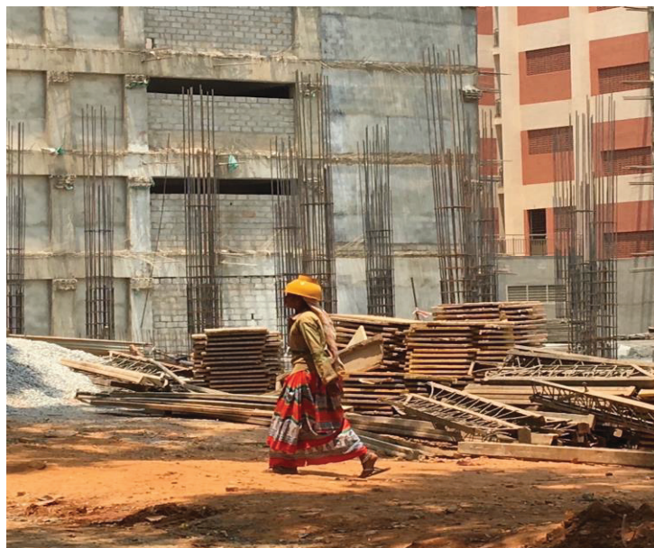
Figure 3. Female worker on Thimmaiah campus site
