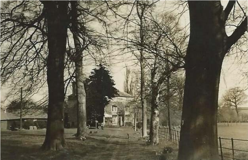
Figure 4. The Avenue in the 1930s
